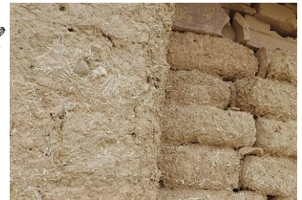
Straw and mud construction.
