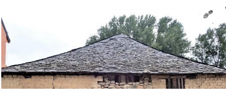
See how they tile a roof in this area.
